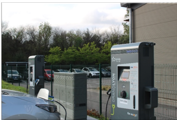
Grand Lyon - borne recharge KEYWATT® 24kW - charge à destination © IZIVIA
